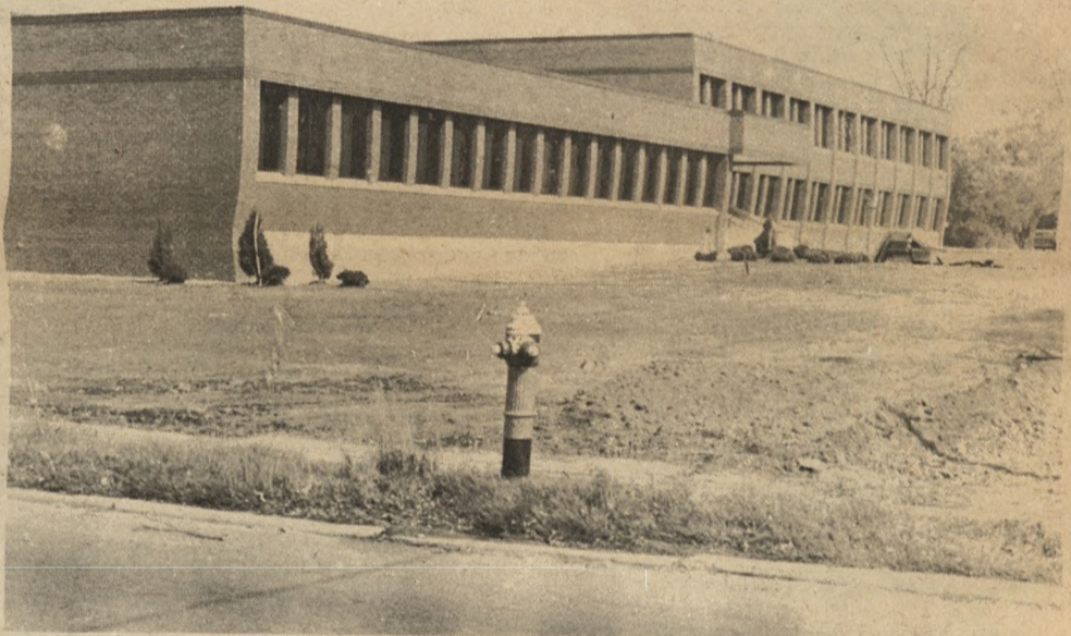
View of new county building from east
