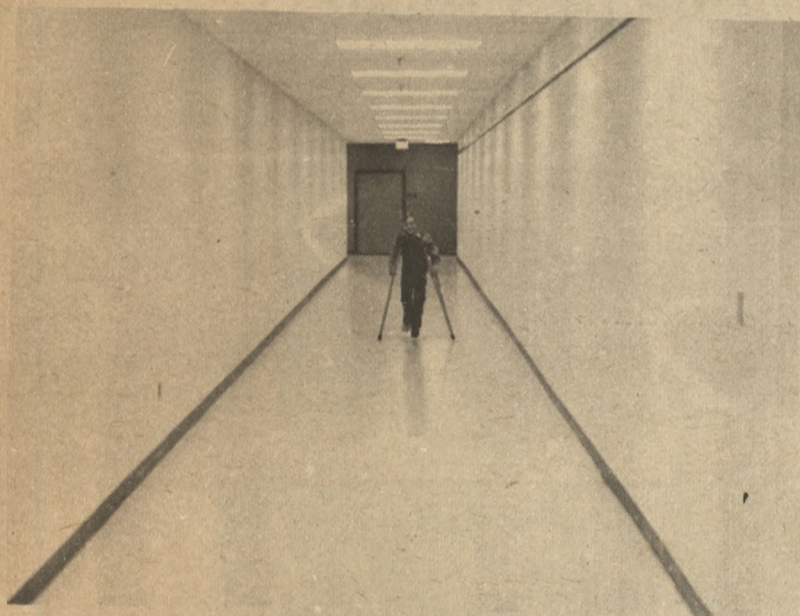
Vinyl covering protects walls in hallways. Most classrooms are carpeted
