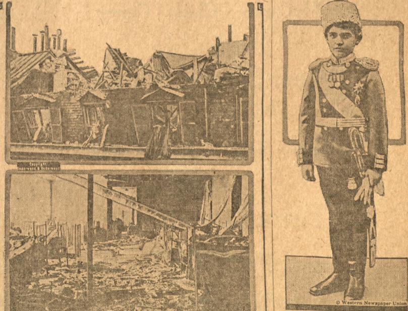
The upper photograph shows a view of several of the houses which were wrecked by the bombs dropped by the Germans. These places of "military importance" to the Germans were the homes of the people who live in the poorer section of Paris. The lower photograph shows the results of bombs dropped on the dormitory of a children's hospital, which fortunately had been vacated in time by the 200 children, and none were injured there. The building is a mass of wreckage. If the children had not been removed doubtless every one of them would have been killed.
