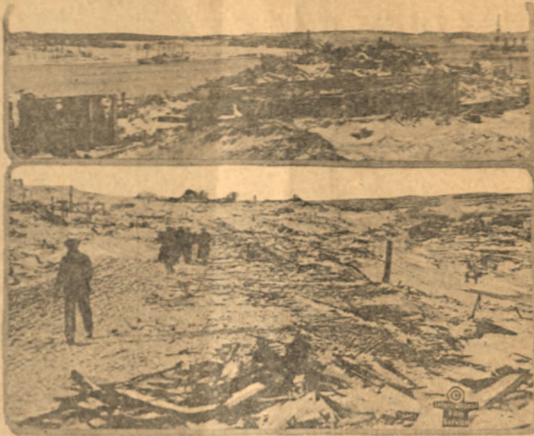
Above, the ruins of the Richmond railway station and docks near which occurred the explosion of a French ammunition ship that wrought such devastation in Halifax and its suburbs. Below, a view along Barrington street where every residence was burned to the ground.
