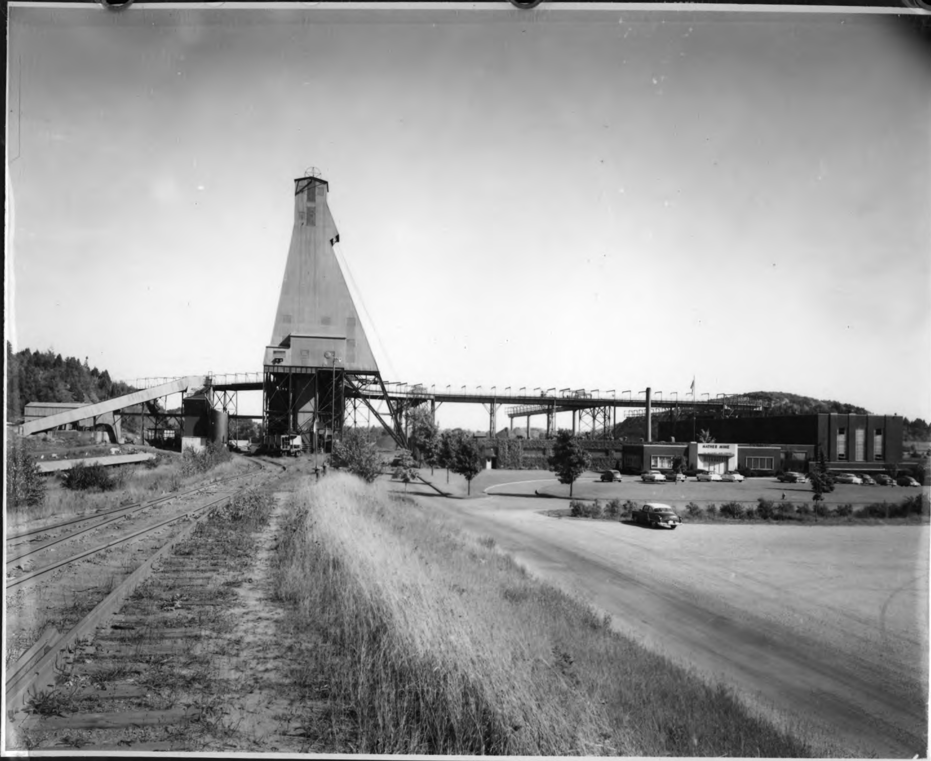
Mather Mine, "A" Shaft Surface Plant (Looking East)
