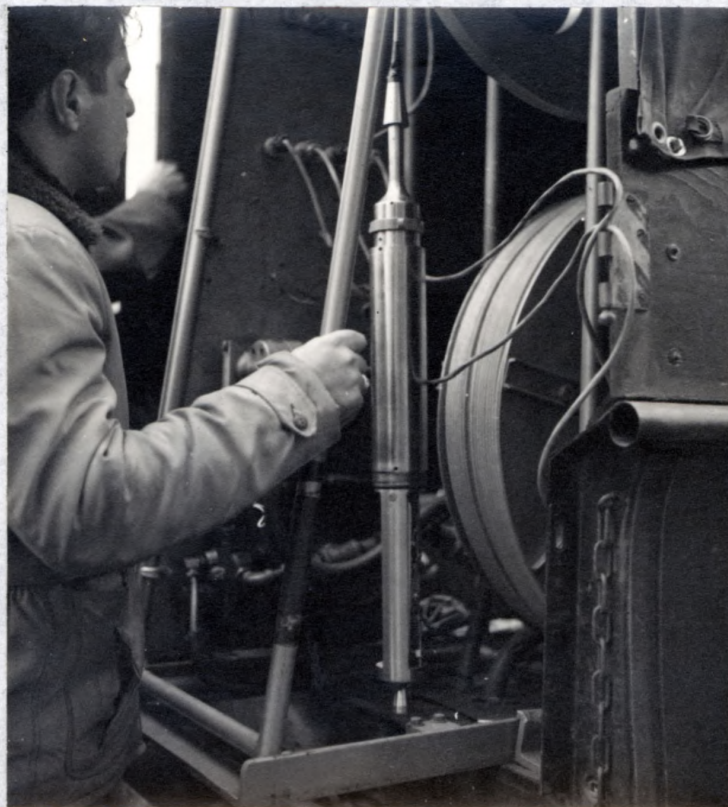
View of Borehole Camera
