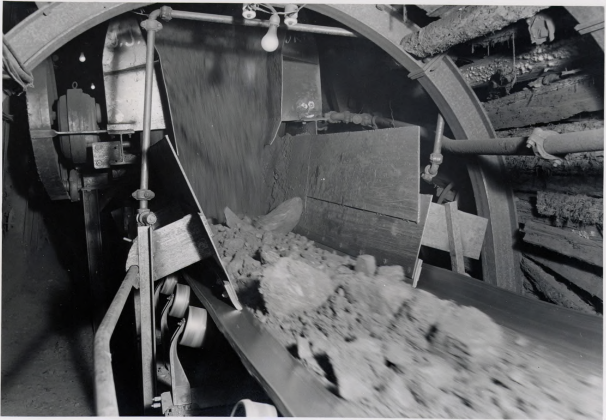
Loading point of conveyor belt located on the -875 sub-level above the 7th Level.
