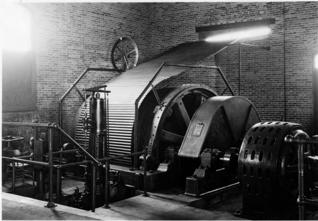
Plate No. 204 - Cage Hoist & Motor - Maas Mine
