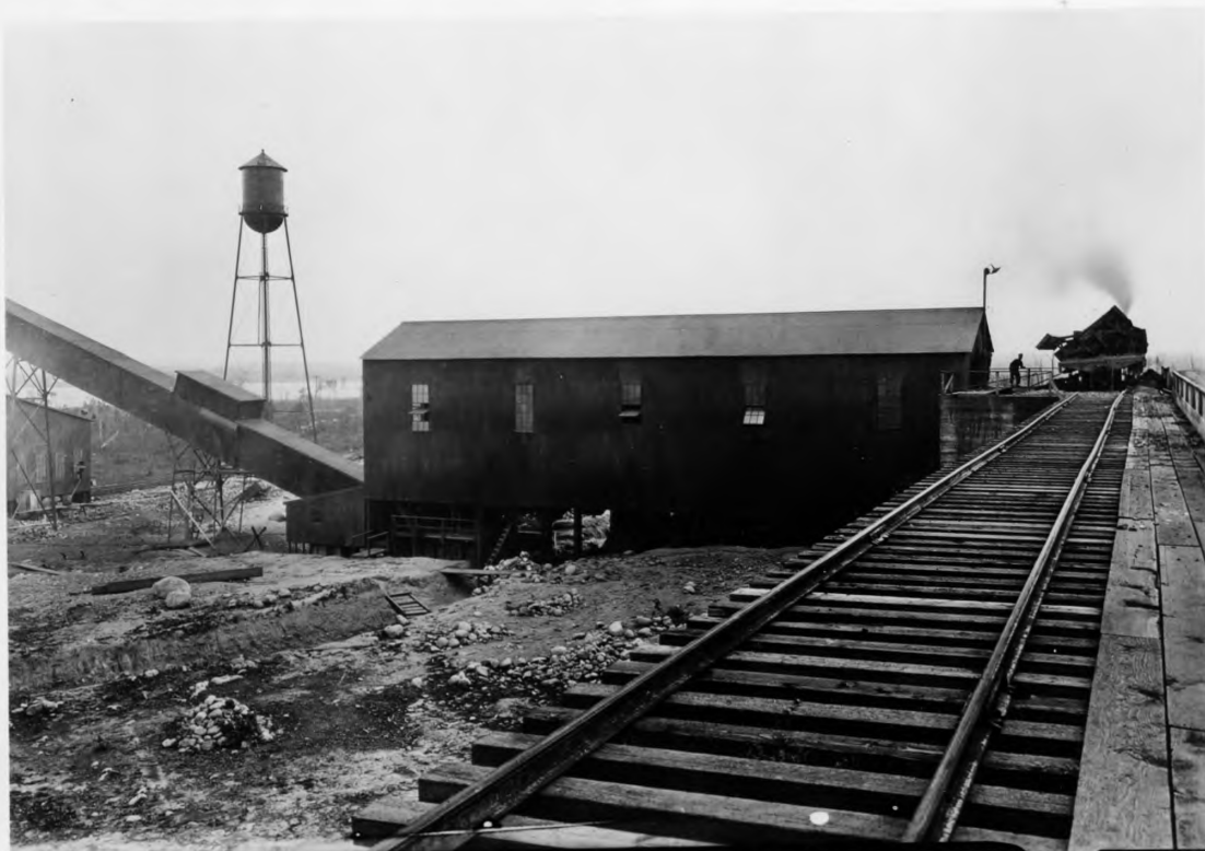
Plate No. 214 - Crusher Bldg. at Washing Plant - Hill-Trumbull Mine
