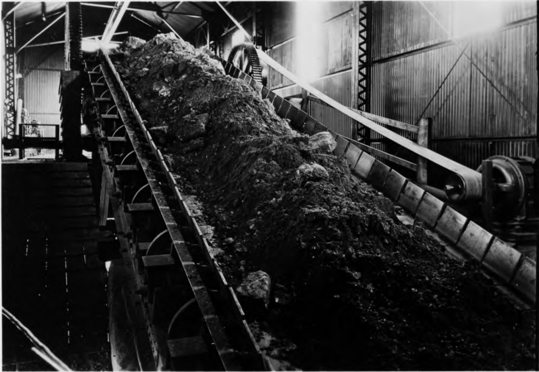
Plate No. 215 - Pan Conveyor - Hill-Trumbull Washing Plant
