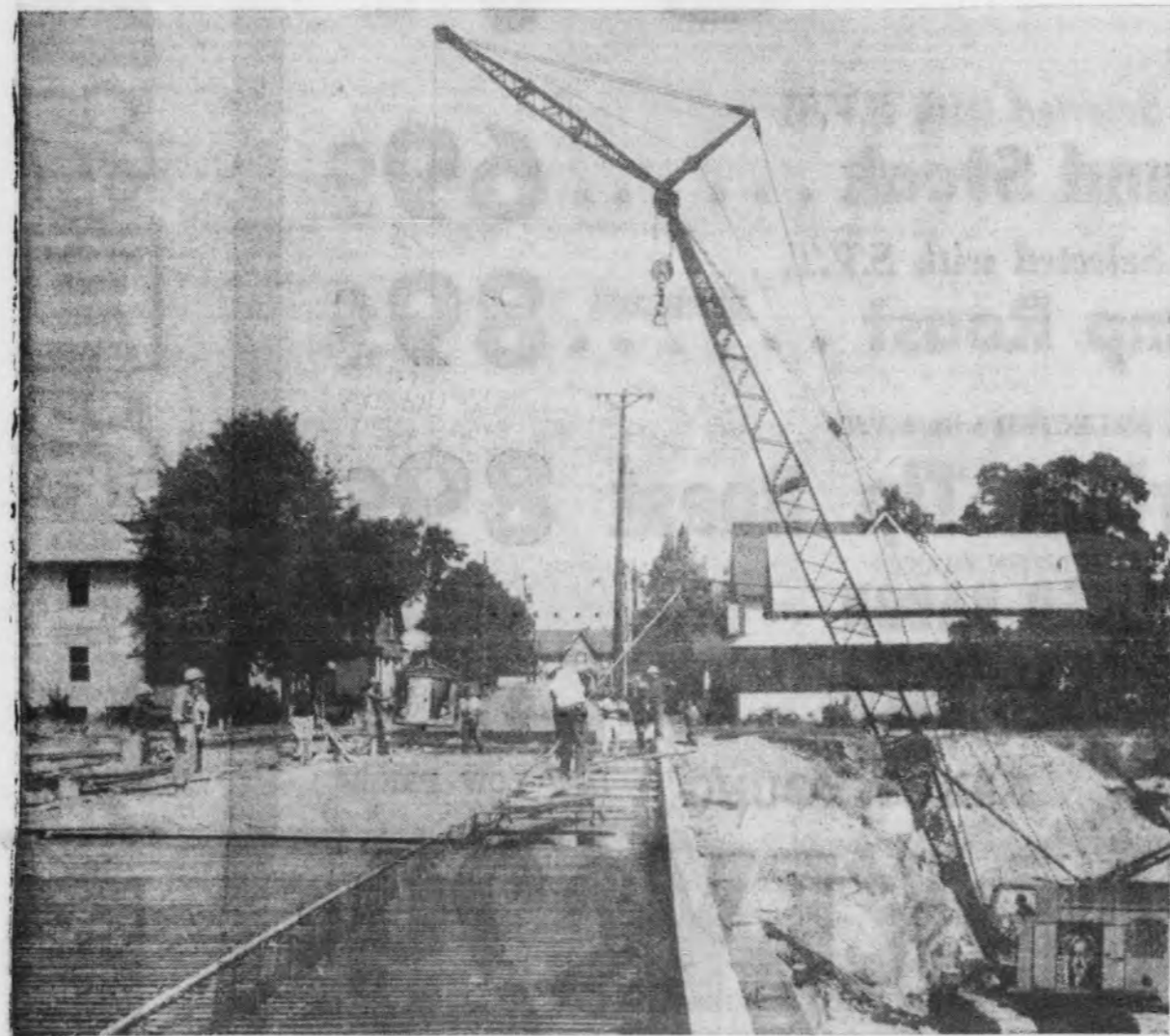
Rapid progress is being made on the construction of the overpasses on the U.S. 41 and M-28 relocation in Marquette. These photos show the work at the Champion St. overpass as it appeared yesterday afternoon. Above is an overall view of the overpass, with a huge crane being used to lift some material into place. Below, the crane is used to place the cement for the pavement on the bridge itself. Above, right, crews of the Bacco Construction Co., Iron Mountain, the general contractor for the work, are smoothing out the concrete on
