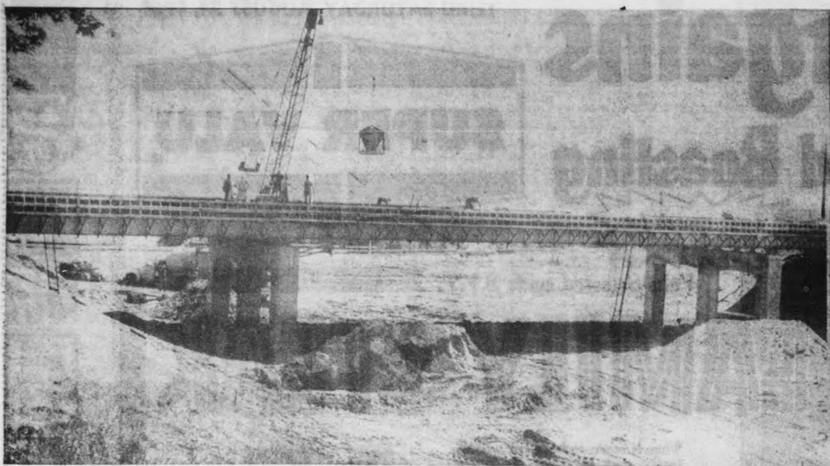
Rapid progress is being made on the construction of the overpasses on the U.S. 41 and M-28 relocation in Marquette. These photos show the work at the Champion St. overpass as it appeared yesterday afternoon. Above is an overall view of the overpass, with a huge crane being used to lift some material into place. Below, the crane is used to place the cement for the pavement on the bridge itself. Above, right, crews of the Bacco Construction Co., Iron Mountain, the general contractor for the work, are smoothing out the concrete on
