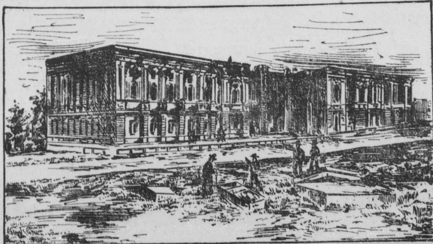
RUINS OF BURNED BUILDING IN 1814.
