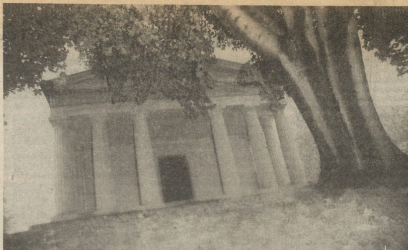
The Mausoleum was just one of the contributions Louis Kaufman made to the Marquette area. (Andy Gregg photo)
