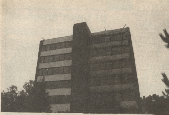
The Cohodas building went through several changes during the summer. Dow Chemical of Midland was responsible for all the work done to replace the masonry. At one point the building was even covered with pale blue and yellow panels before the final facade was in place. The facelift is scheduled to be complete in the first week of October. Final touches will include dark bronze window sills. (George Hannemann photo)
