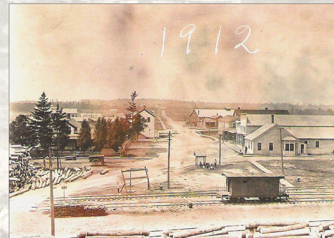
Looking north; Lumber Company Office is the closest building on the right side of photo.
