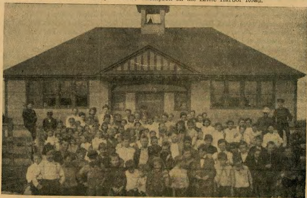
The school building presently in use in Thompson township is shown here in early years after its construction, with a class in the early 1900s standing before it. The old wood building is rated not fire-safe and efforts are underway to build a new school.
