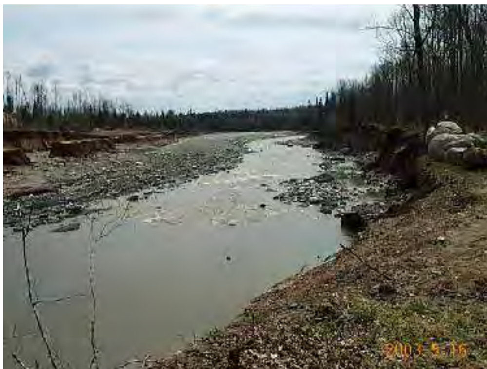
Figure 5. Looking downstream from the former location of the fuse plug towards Dead River; taken on May 16, 2003 (Source: FERC, 2003b)
