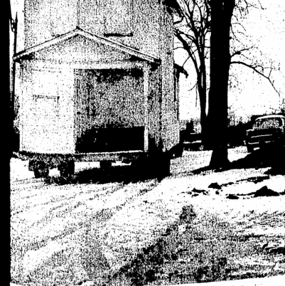
ON THE MOVE—A king-size house trailer? No, it's the Post House Museum on wheels, just arrived at its new location adjacent to the old water tower. The building is now secured on a new foundation, and will be opened in the spring as a major tourist attraction in the community.
