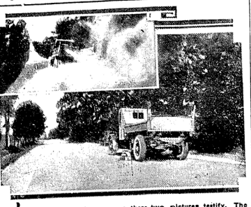
DUSTY highways are dangerous as these two pictures testify. The upper photo shows a truck with grader operating on a gravel road which never has been treated with calcium chloride. Note the clouds which never have been treated with calcium chloride. Note the clouds which never have been treated with calcium chloride. Note the clouds which never have been treated with calcium chloride.
