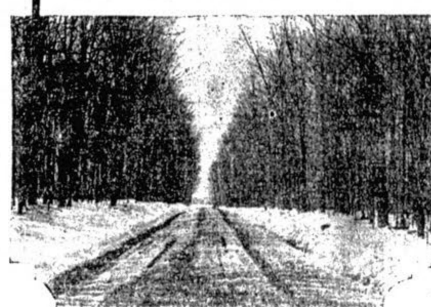
Log houses were built to house the members of the "Utopian Colony" founded near Manistique, Mich., in 1893, as the Hiawatha Village Association. Byers, leader of the movement, induced Mills and Randall to join and work out the colony's scheme of government. The colony in its house (center) still stands. A road cleared by the members, leading across their property, now is a part of M-94.
