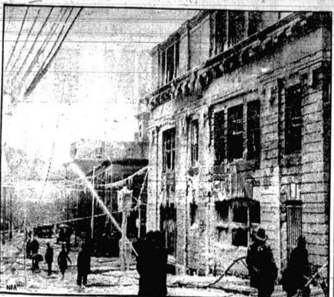
The fame-swept shell of the Wilbur hotel on Main Street, Fall River, is pictured here. Firemen of Fall River and several neighboring cities had to contend with freezing cold as they manned their apparatus. Note how buildings, wires, and street are sheathed with ice in this remarkable view, taken while the fire still was burning.
