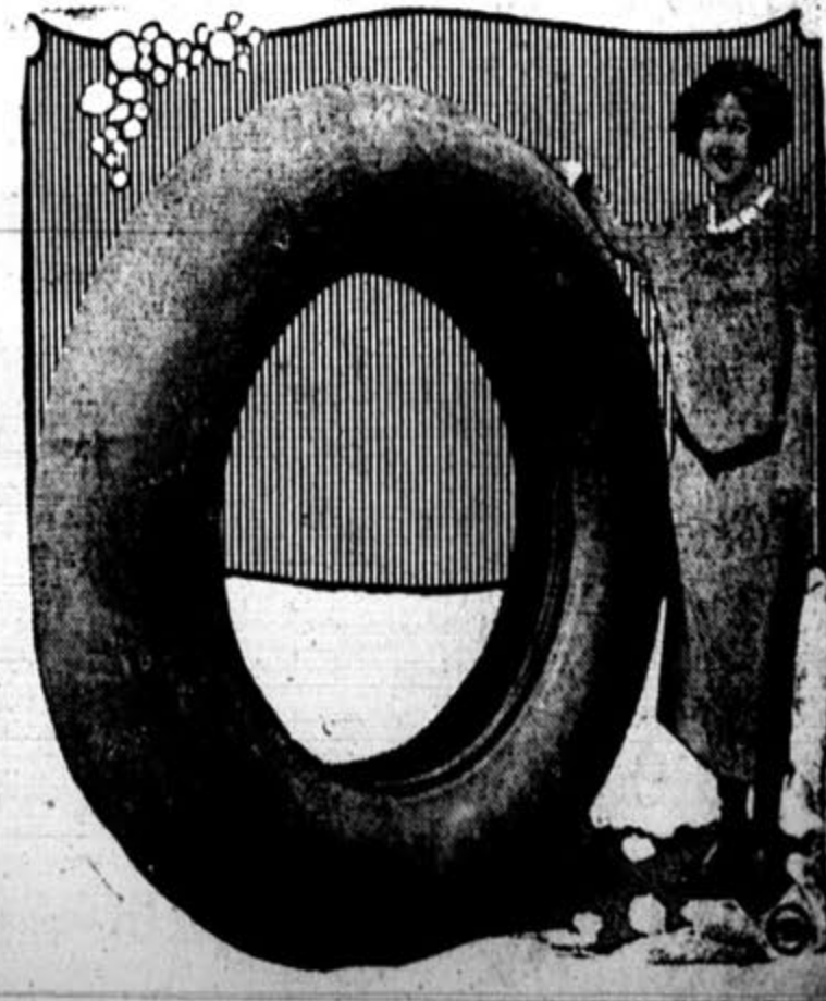
HERE'S LARGEST PNEUMATIC TIRE —Uncle Sam's air service again excels—this time in the size of airplane tires. The young lady is just as tall as the tire, which will be used on a special type of airplane now being perfected. It is a 64 by 14-inch balloon tire cord and will sustain a load of 20,000 pounds at an inflation pressure of 75 pounds. The tire was made at Akron.
