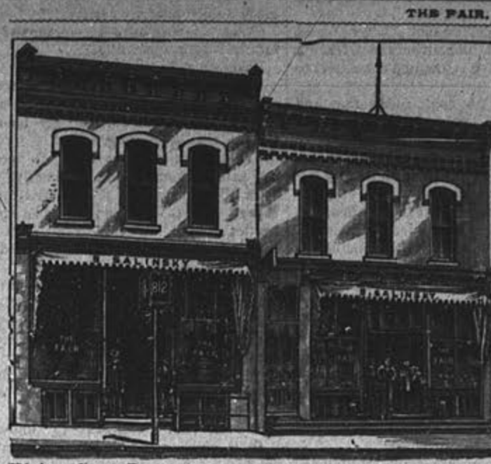
This Cut Represents the Fair Building. 812 AND 814 LUDINGTON STREET.
