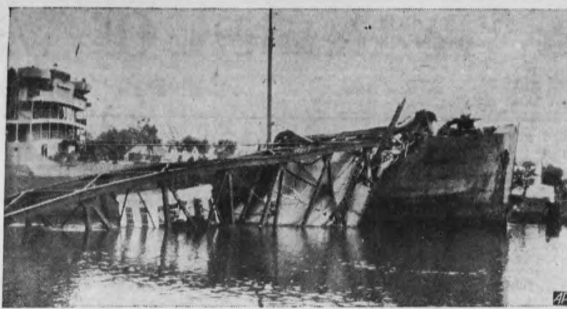
TANKER KNOCKS DOWN BIG BRIDGE —Wreckage of the 226-foot highway drawbridge over the Chesapeake and Delaware canal, important inland waterway, lies across the bow of the oil tanker which crashed into the structure near Chesapeake City, Md. Both of the 200-foot towers on which the span was swung fell into the canal, running between the Delaware river and Chesapeake bay.
