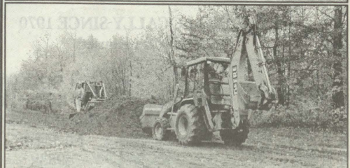
Grading and leveling Harju Rd. is progressing.
