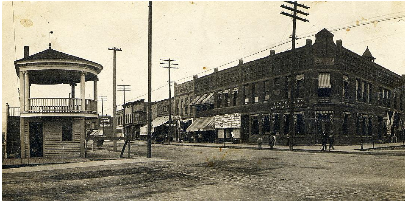
East Side of the 200 Block of South Stephenson Avenue with Band Stand/Police Station, Iron Mountain, ca. 1911: This postcard view, postmarked March 30, 1911, shows the northeast corner of South Stephenson Avenue and East Ludington Street. Note the raised band shell on the northwest corner with the city's police quarters housed below and the brick pedestrian crosswalk. The First National Bank occupied about one-half of the Wood Block at this time. [William John Cummings]
