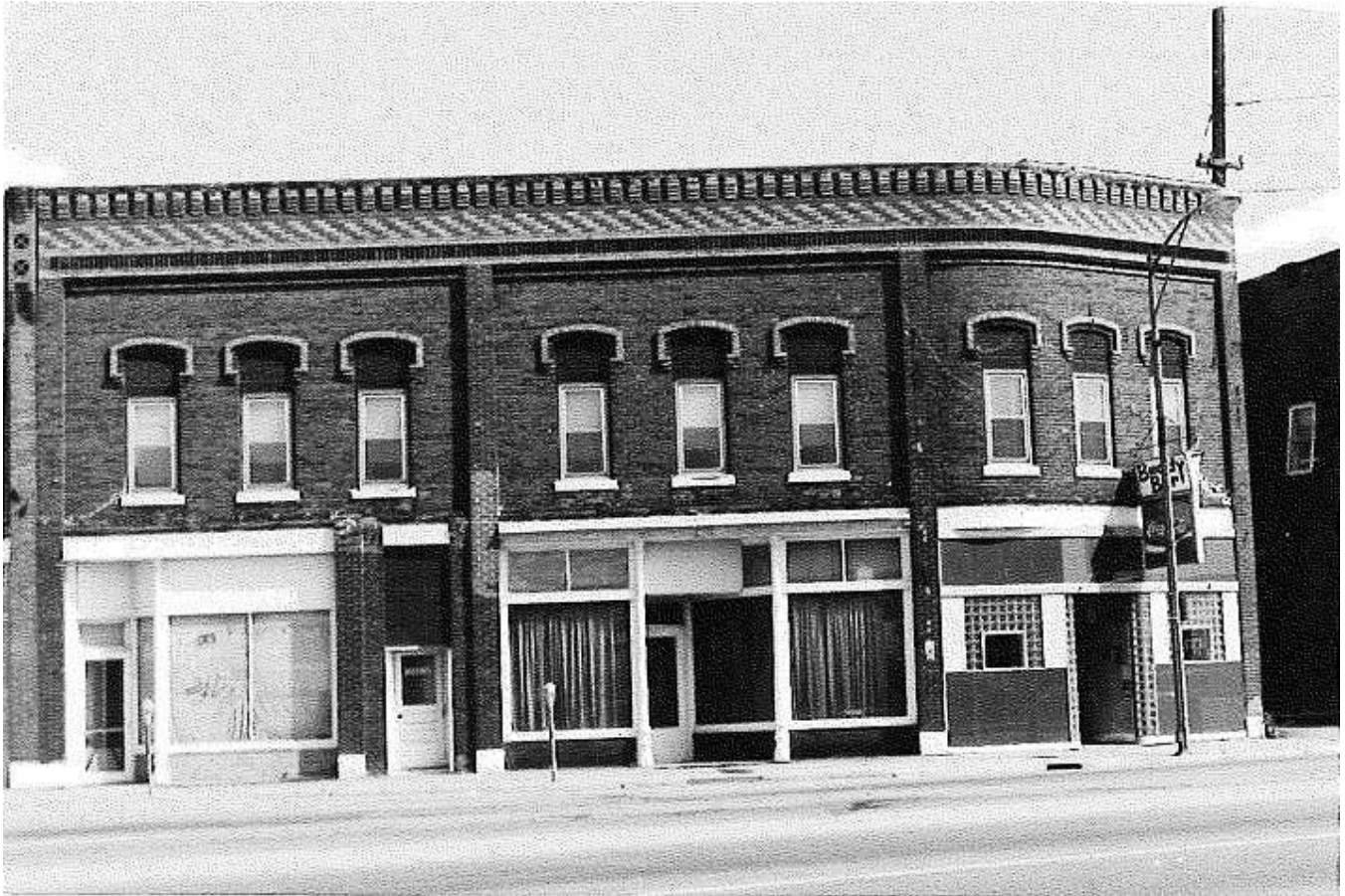
South Half of the East Side of the 100 Block of South Stephenson Avenue, Iron Mountain, 1975: Taken during a State of Michigan Survey in 1975, the south half of the double building located on the 100 Block of South Stephenson Avenue shows 115 South Stephenson Avenue and other addresses before the remodeling was done for the Lonely Bull, Geline's Rib Cage and Fontana's Supper Club. [State of Michigan]
