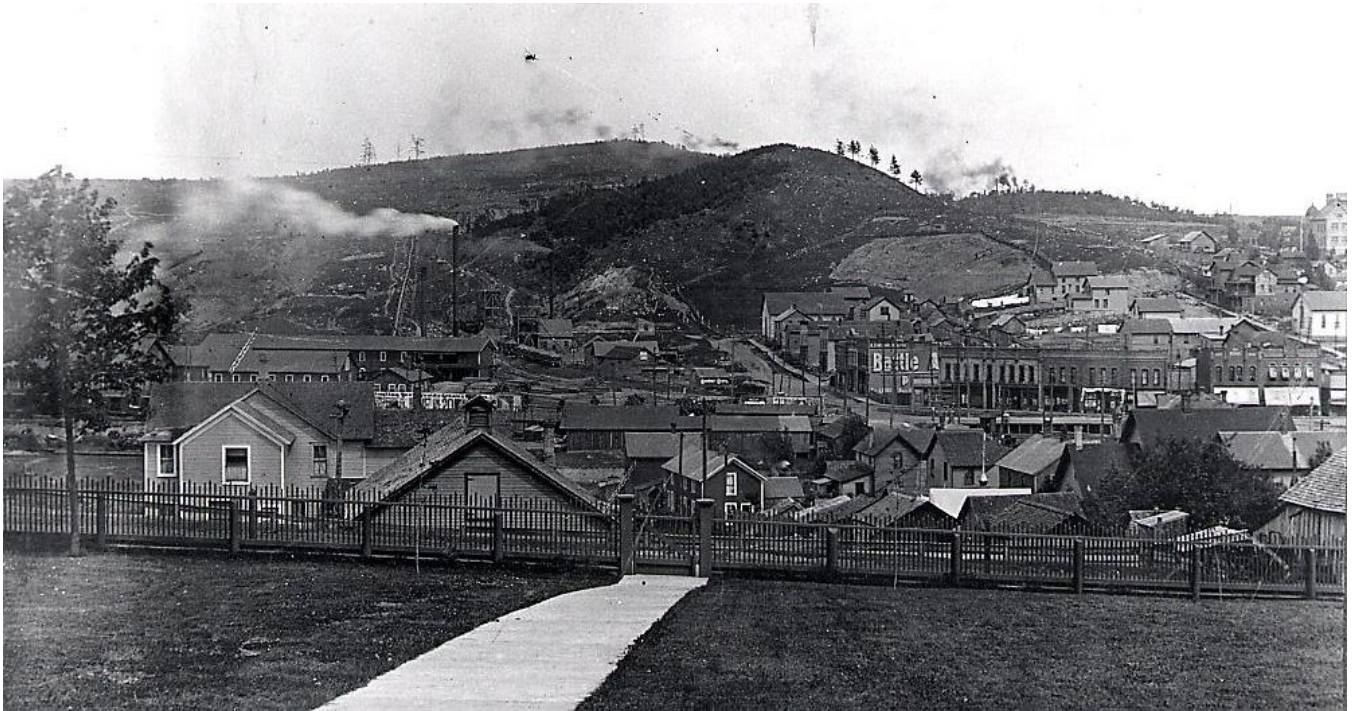
Chapin Mine Shops and 100 Block of South Stephenson Avenue, Iron Mountain, ca. 1910-1915: Probably taken in about 1910-1915 from the Ludington Mine Location looking east, the stores on the 100 block of South Stephenson Avenue are visible, as well as Pewabic Hill and Millie Hill with the Nelson P. Hulst High School barely visible at the far right. [Menominee Range Historical Museum]
