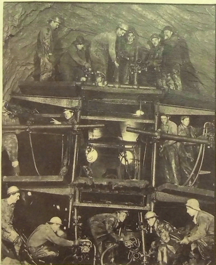
Drill Jumbo at one of the four headings.
